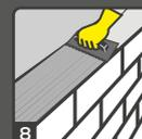
Put well-mixed mortar on the block with the help of trowel spread mortar uniformly on the unit for the specified bed thickness.
