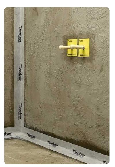
2K elastomeric waterproofing coat for cementitious substrate weber waterseal 321
